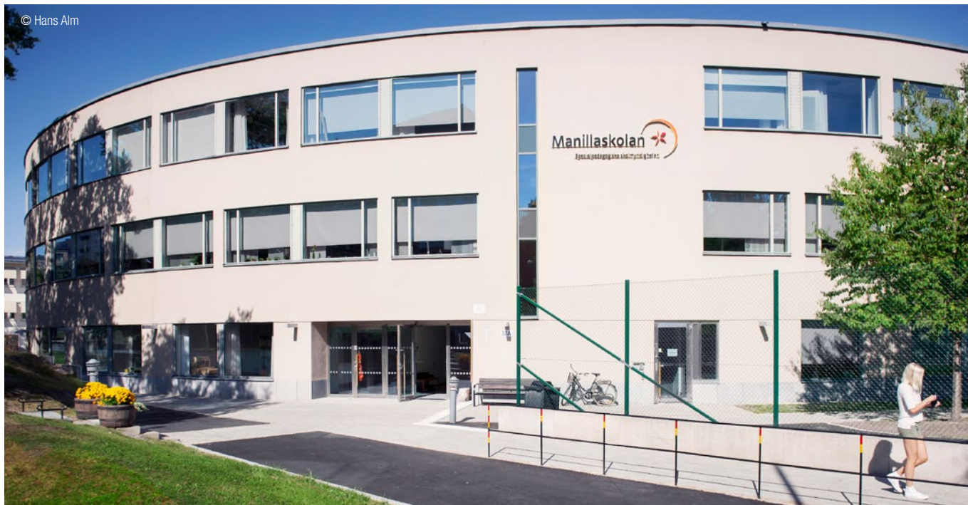
Die Wireless-BACnet-Technologie reduzierte die Installationszeit um 65 %. Wireless BACnet technology reduced the installation time with 65%.
