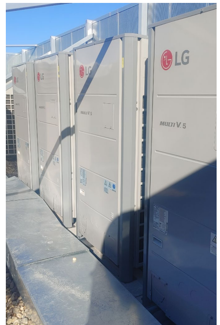
Multi V 5 Outdoor Units. © LG Electronics
