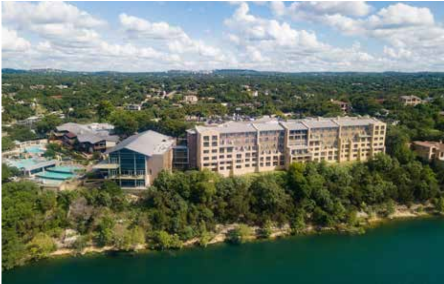
Luxury Texas resort enhances guest comfort with Wireless HVAC Retrofit. Luxusresort in Texas verbessert Gästekomfort durch drahtloses HKL-Retrofit.
